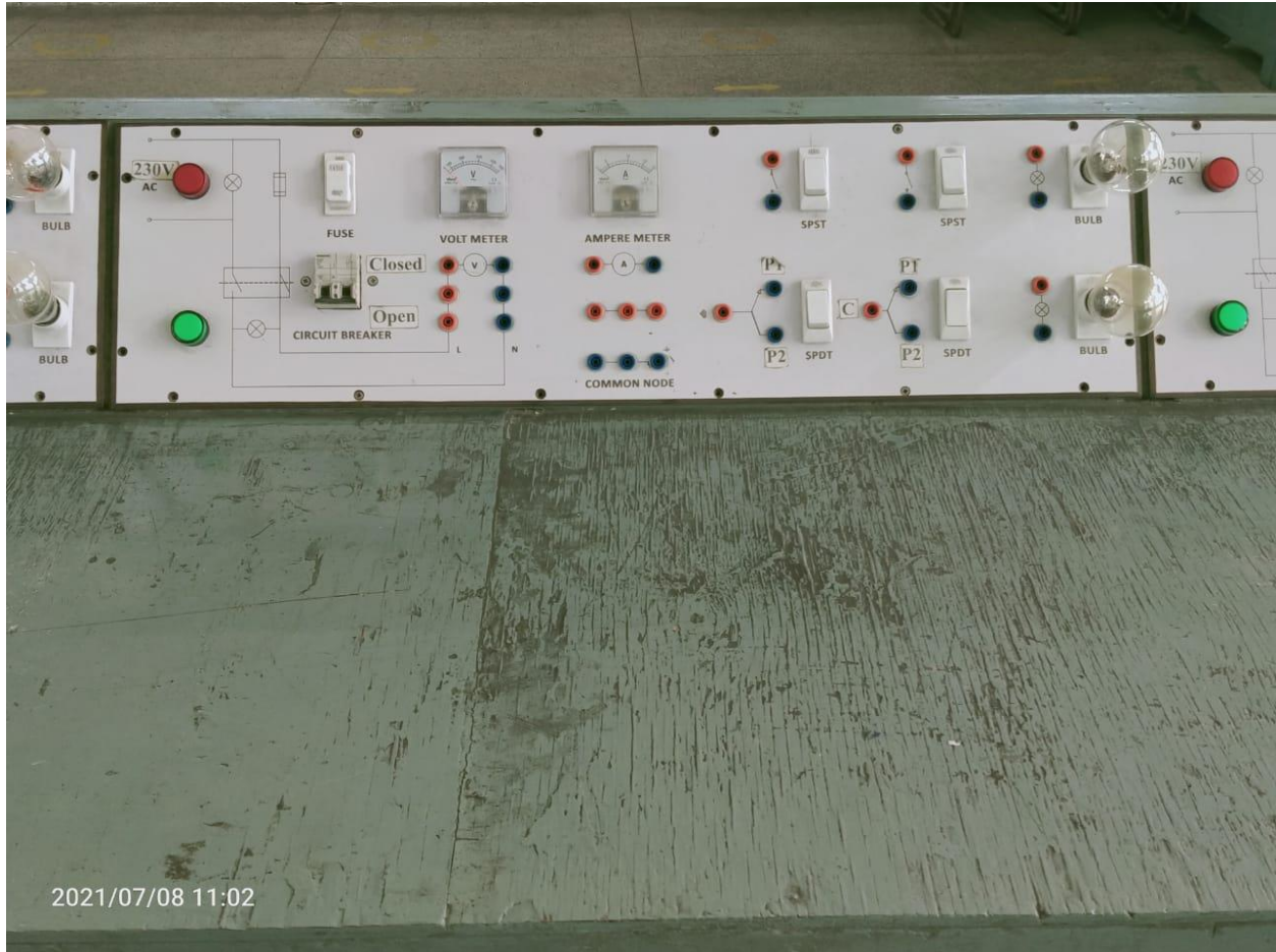
Wiring Panel Working Table
