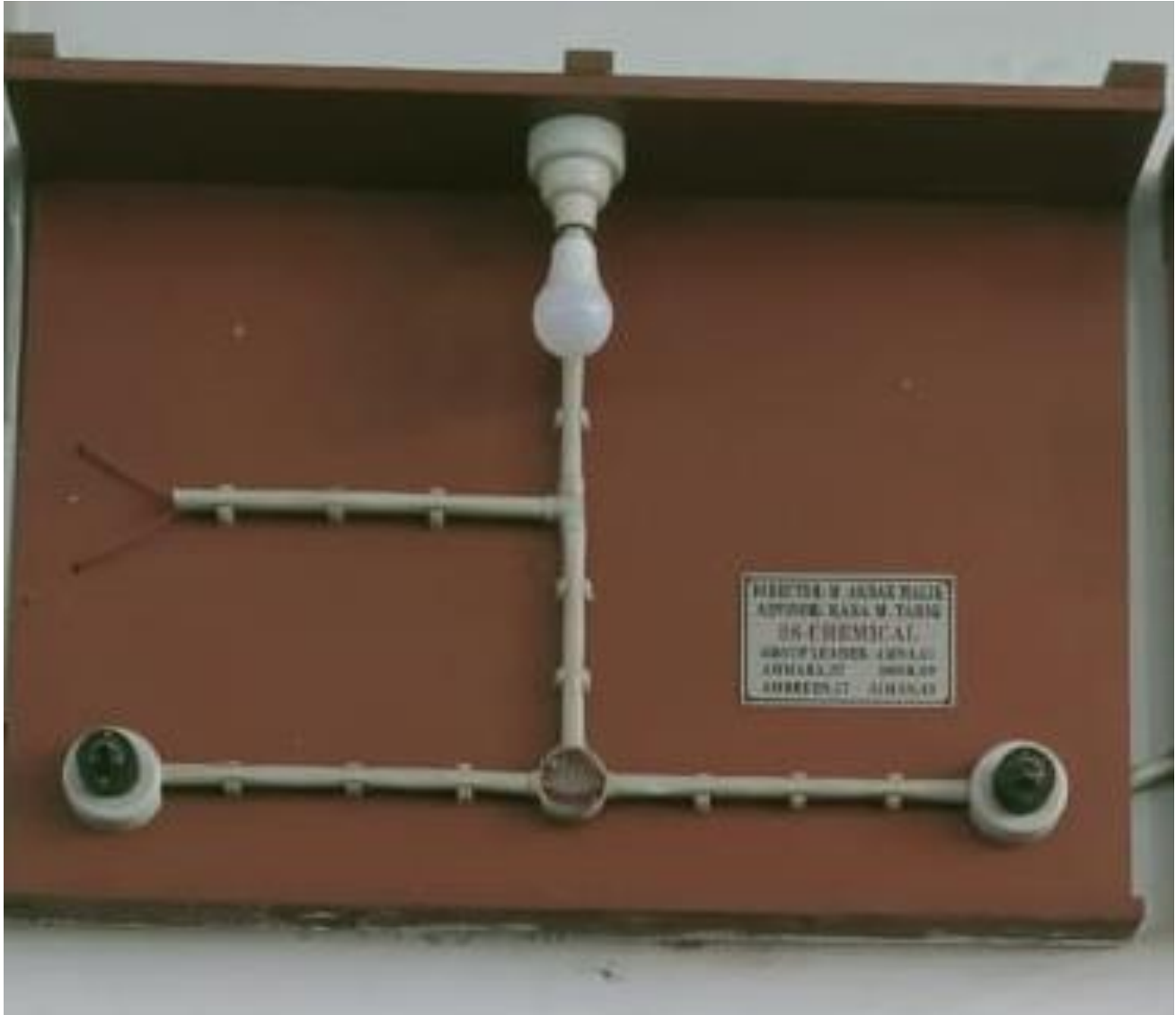
PVC Exposed Conduit Wiring Demonstration
