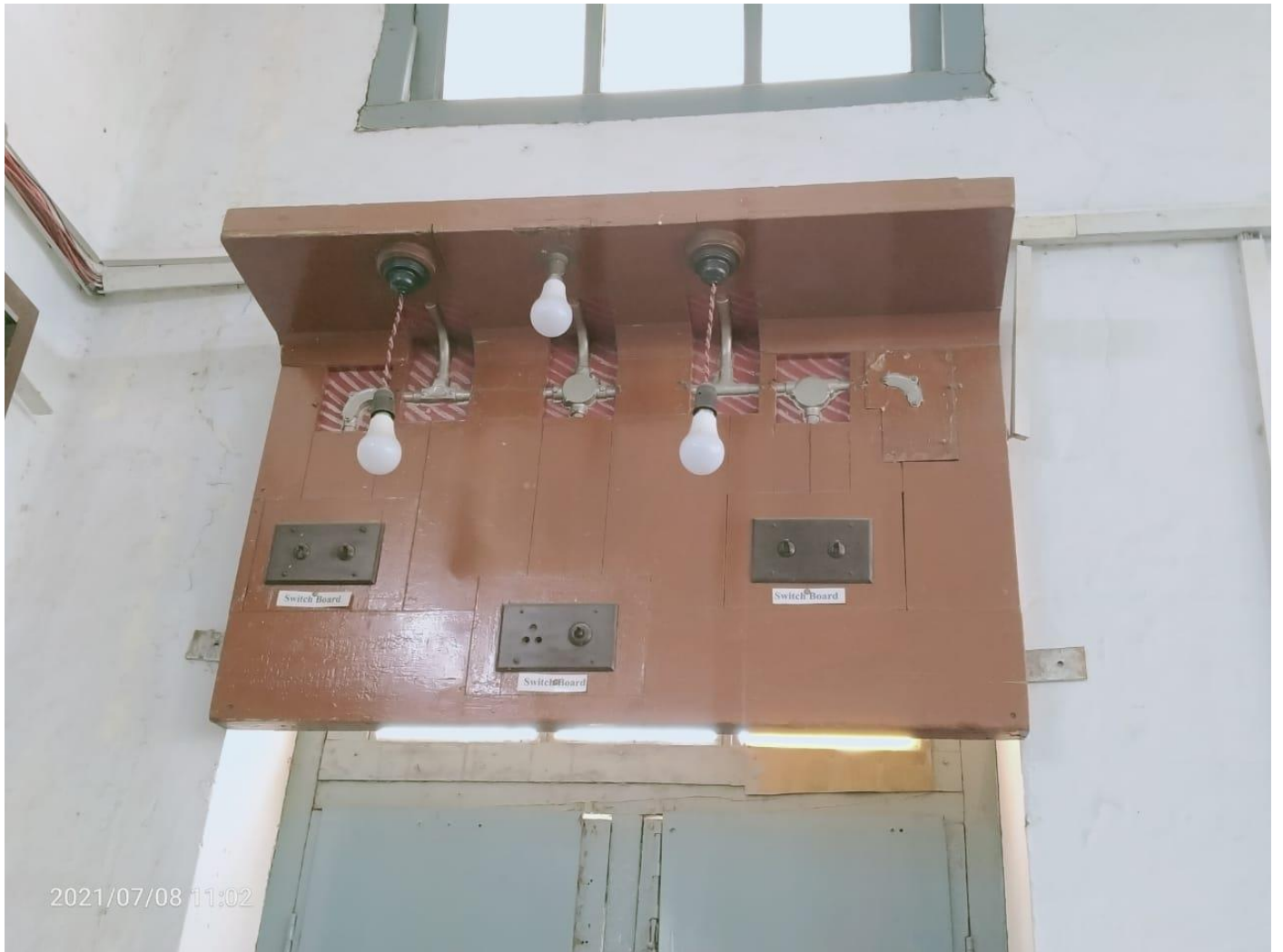
Concealed Conduit Wiring Demonstration
